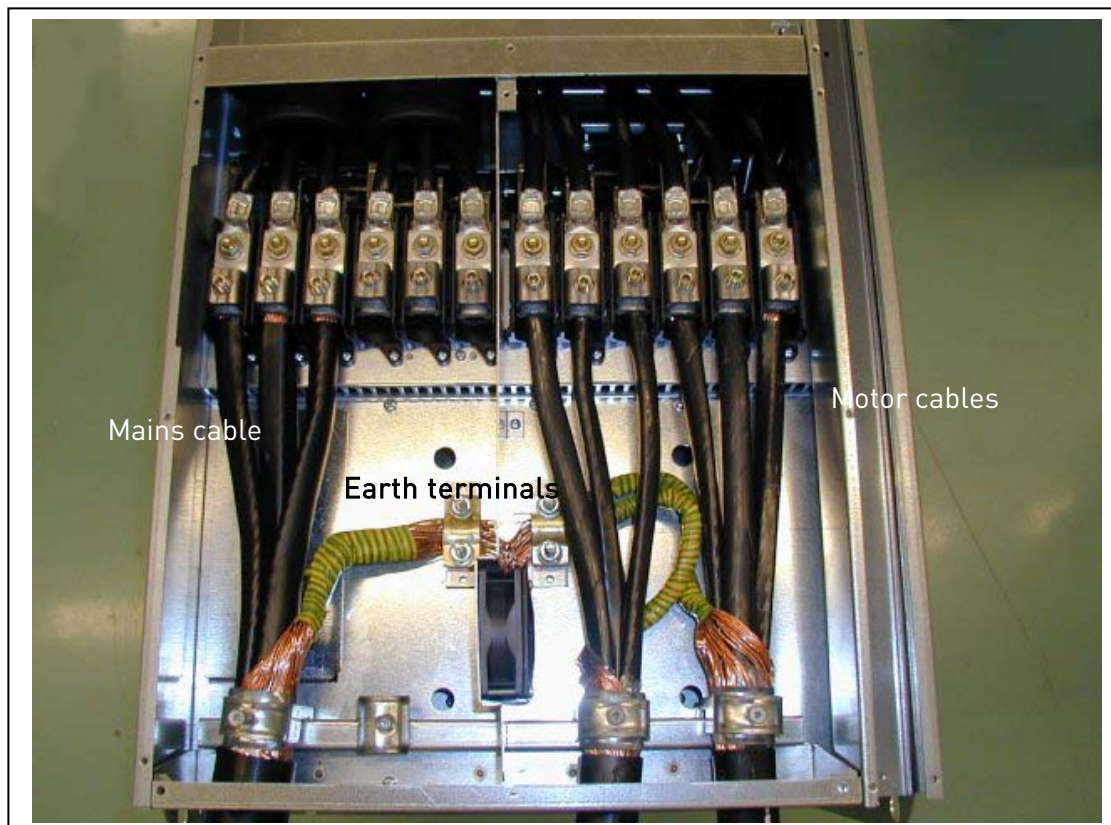
Figure 6-22. Cable installation in Vacon NX5/P, FR9
