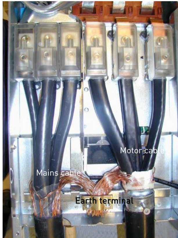
Figure 6-18. Cable installation in Vacon NXS/P, FR8
