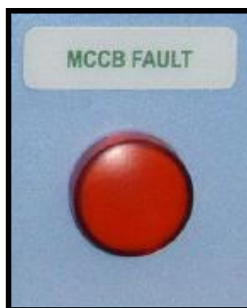
Figure 7-5. MCCB FAULT indicator
