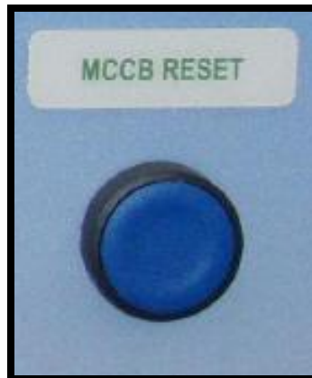
Figure 7-6. MCCB Reset push-button (-S11)
